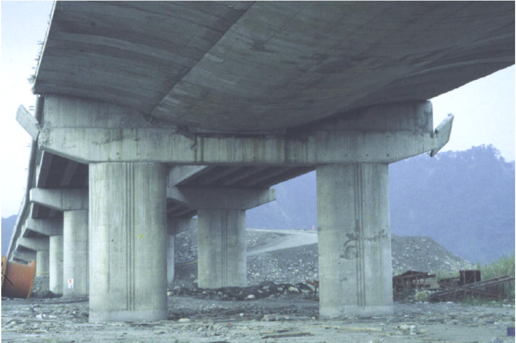
Cable-Stayed Bridge, 1999 Chi-Chi Eq. (M.O. Eberhard)
