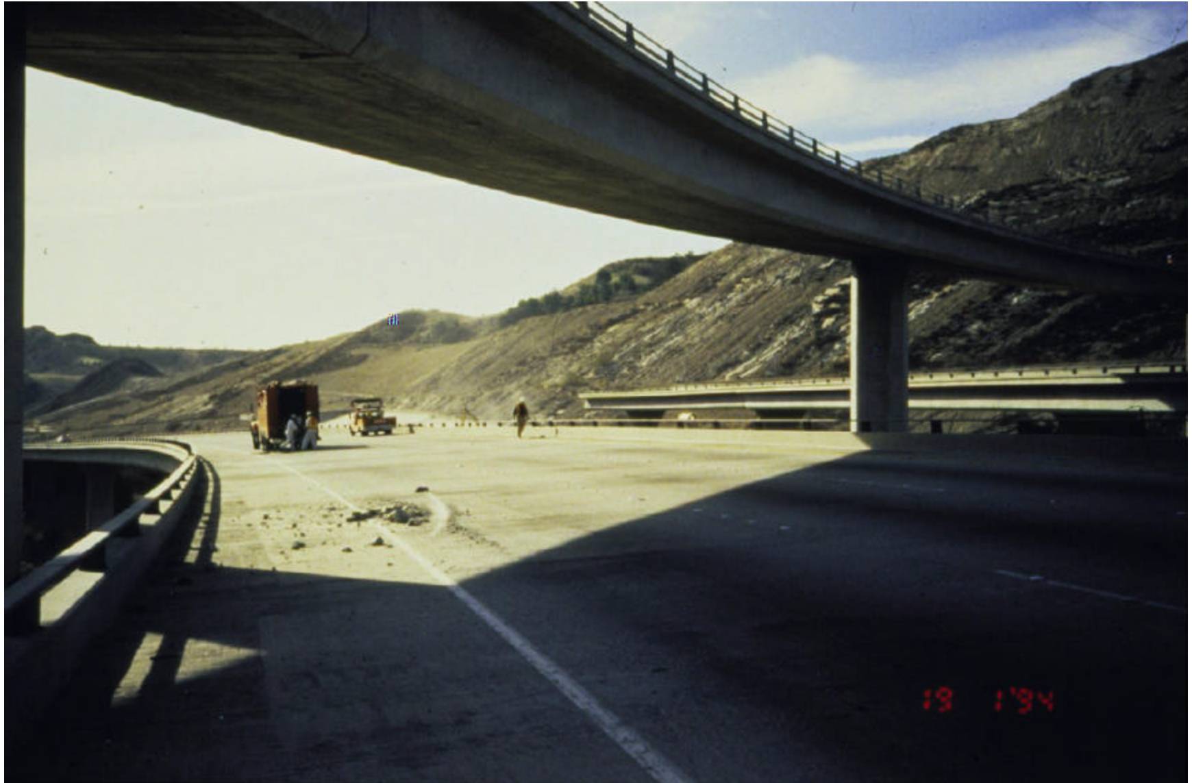
I5-14,1994 Northridge Earthquake (M.O. Eberhard)
