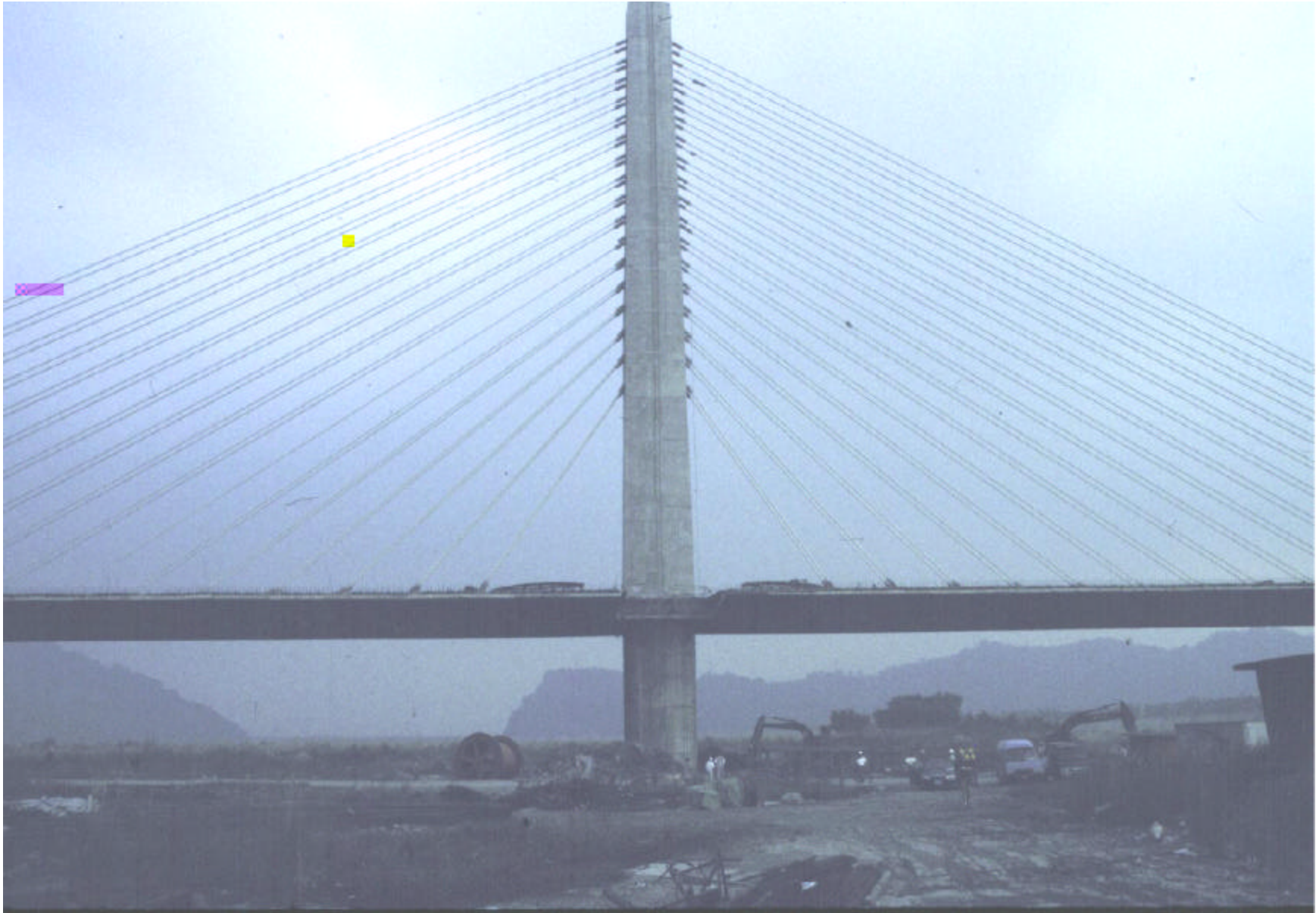
Cable-Stayed Bridge, 1999 Chi-Chi Eq. (M.O. Eberhard)
