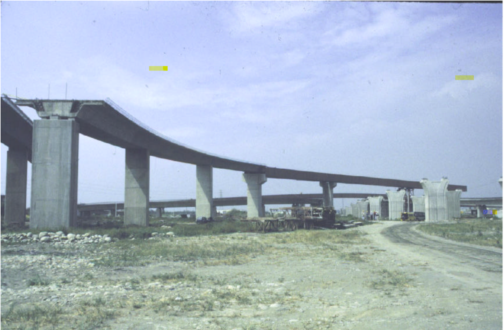
1-3 Expressway Link, 1999 Chi-Chi Eq. (M.O. Eberhard)
