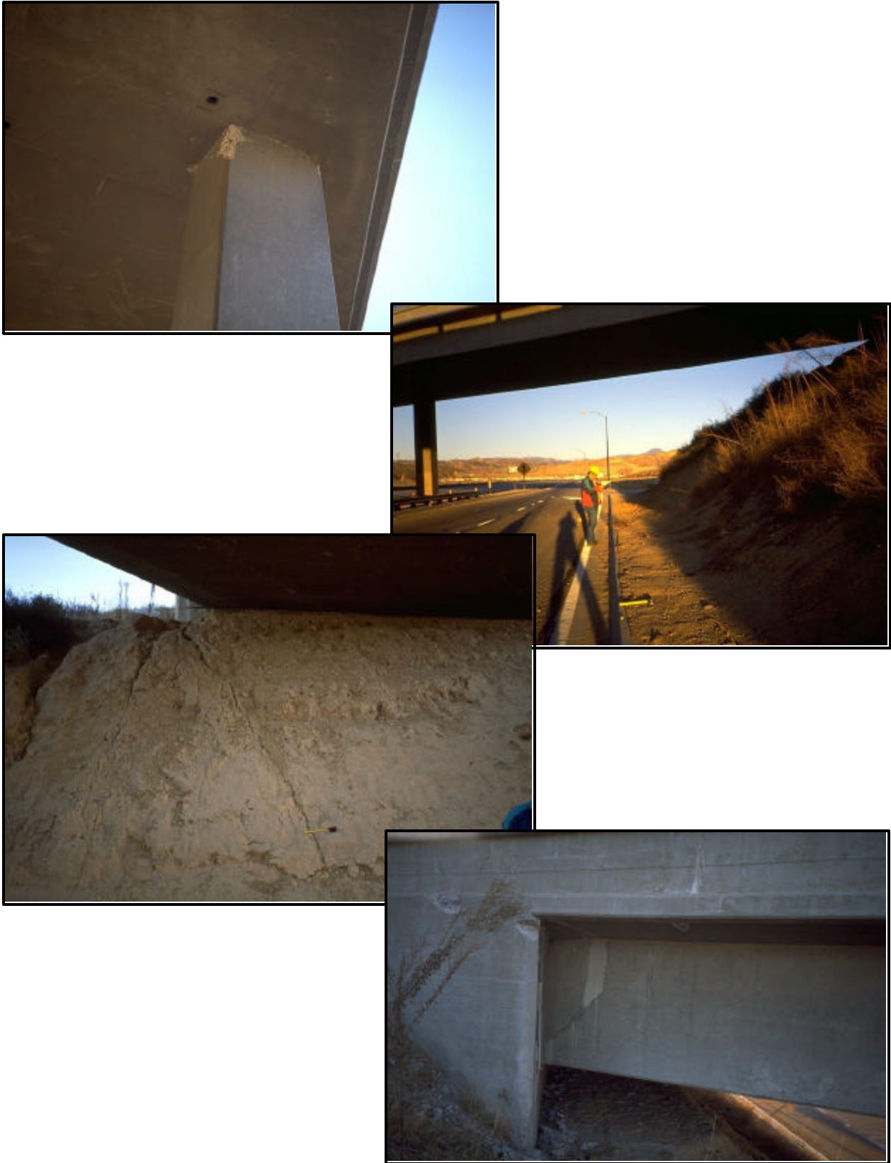
FIGURE 8.22 Different views of the superstructure of the bridge (11)
