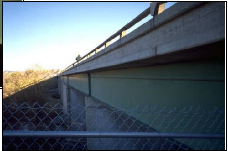
FIGURE 8.3 Different views of bridge superstructure (11)
