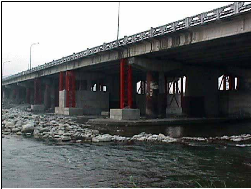
FIGURE 7.4 Another view of temporary shoring after Taiwan Earthquake 1999 (11)
