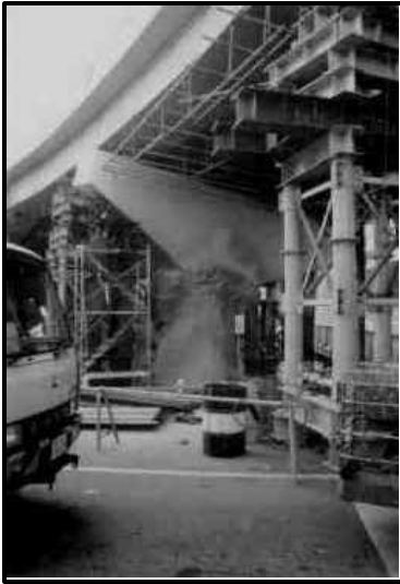
FIGURE 7.8 View of temporary shoring to prevent total collapse of steel bridge (27)
