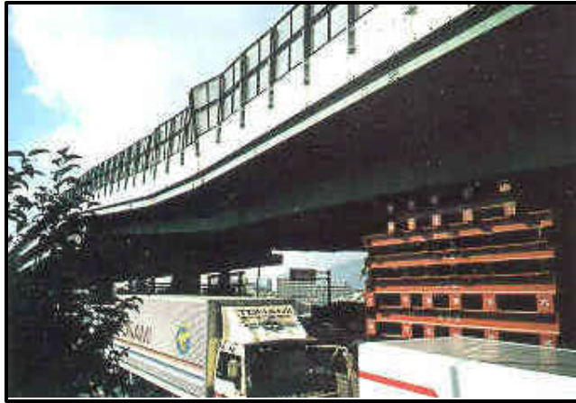
FIGURE 7.5 View of temporary shoring to maintain access after Kobe Earthquake 1995 (27)
