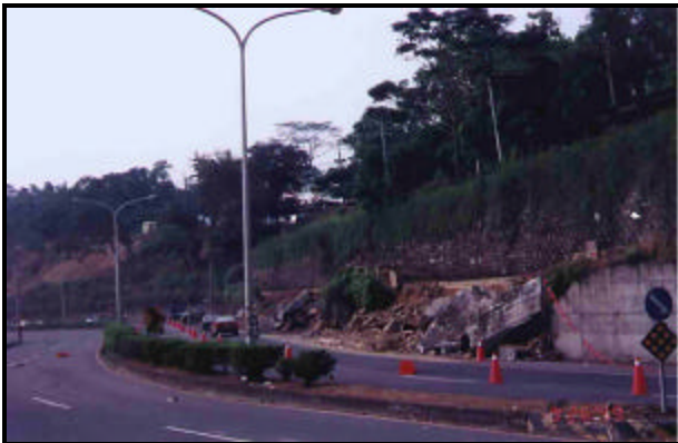
FIGURE 5.78 Retaining wall failure after Taiwan EQ 1999 (26)
