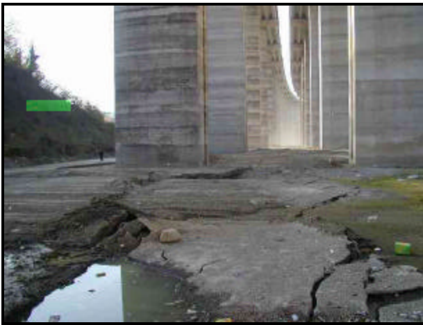
FIGURE 5.84 Soil failure due to the fault movement through RC bridge piers after Duzce EQ 1999 (10)
