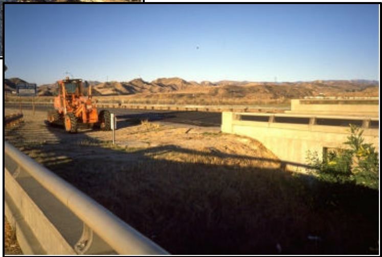
FIGURE 8.24 Different views of the second example bridge (11)
