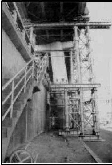
FIGURE 7.11 View of temporary support to prevent total collapse of steel bridge (27)
