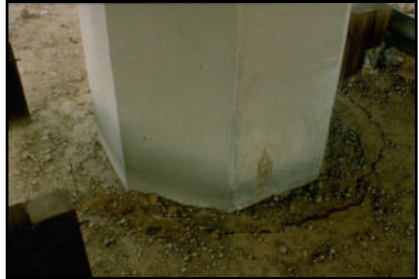
FIGURE 3.43 Disturbed soil at the base of column after Northridge EQ 1994 (11)
