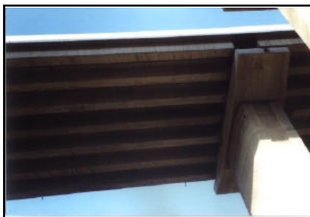
FIGURE 3.16 Longitudinal movement of RC box girders after Duzce EQ 1999 (10)
