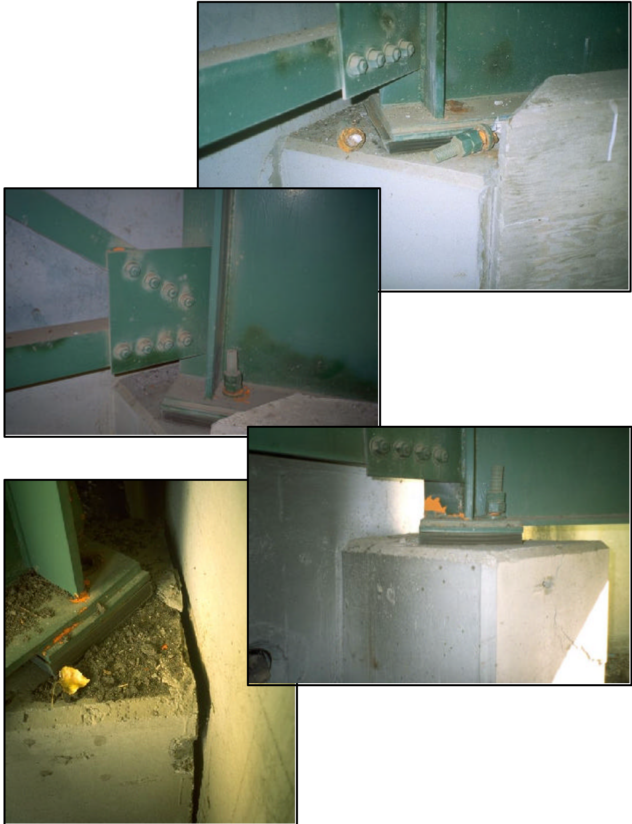
FIGURE 5.7 Damage to the bridge bearings (11)
