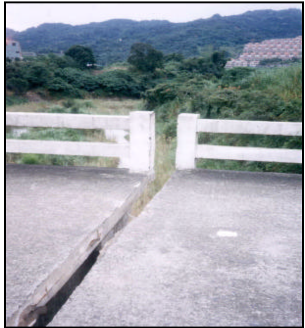
FIGURE 3.11 Excessive longitudinal movement of the bridge deck (15)
