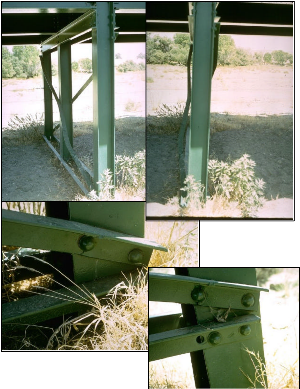
FIGURE 5.12 View of the damaged bridge components (11)
