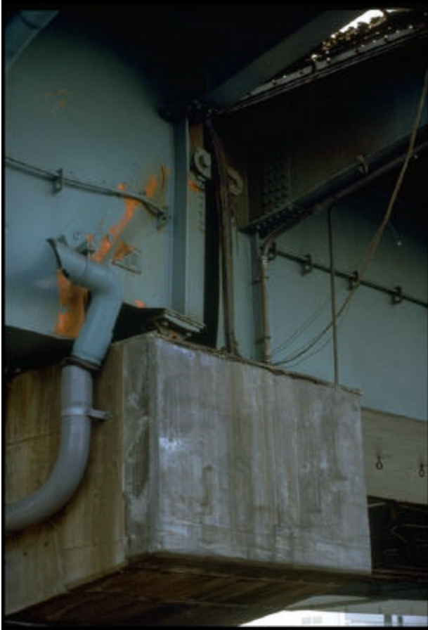
FIGURE 3.63 Buckling in the girder due to pounding (11)
