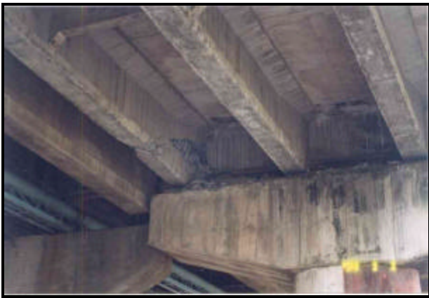
FIGURE 3.68 Shear cracks at the RC bridge girder near support (26)
