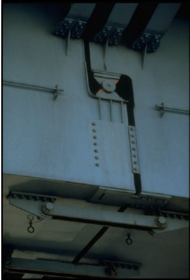
FIGURE 3.59 Yield at pin support (in red color) (11)
