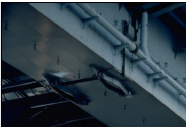
FIGURE 3.85 Buckled seismic restrainers (11)
