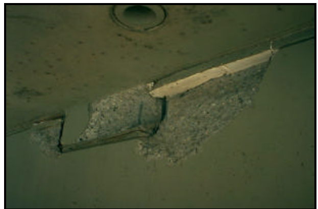
FIGURE 3.30. Shear key failure of a bridge after Northridge Earthquake 1994 (11)
