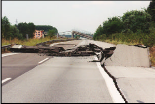
FIGURE 3.4 Collapse of roadway due to fault rupture after Izmit EQ 1999 (10)
