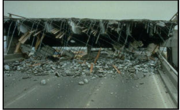
FIGURE 3.7. Failure of a monolithic RC girder bridge after Loma Prieta EQ 1989 (11)
