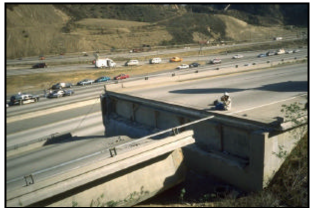
FIGURE 3.9 Collapse of bridge deck after Northridge 1994 (11)
