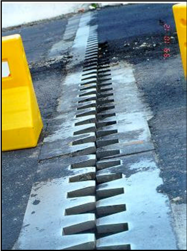
FIGURE 3.18 Excessive movement of expansion joints after Taiwan EQ 1999 (15)
