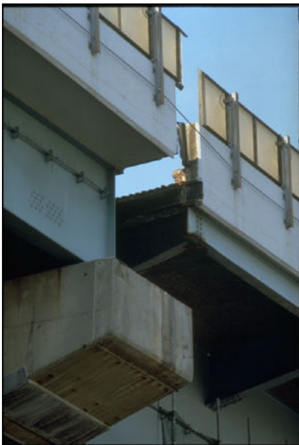
FIGURE 3.13 Excessive longitudinal movement of steel box girder bridge (11)
