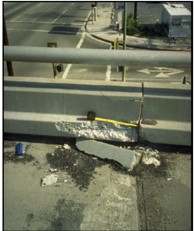
FIGURE 3.44 Barrier cracking after Northridge Earthquake 1994 (11)
