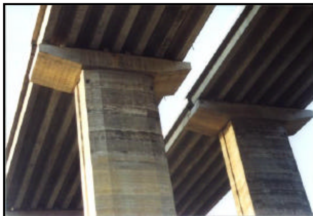
FIGURE 3.15 Lateral movement of prestressed RC box girders (10)
