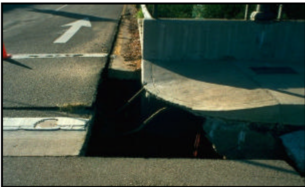
FIGURE 3.47 Collapse of asphalt pavement due to washout after Northridge EQ 1994 (11)
