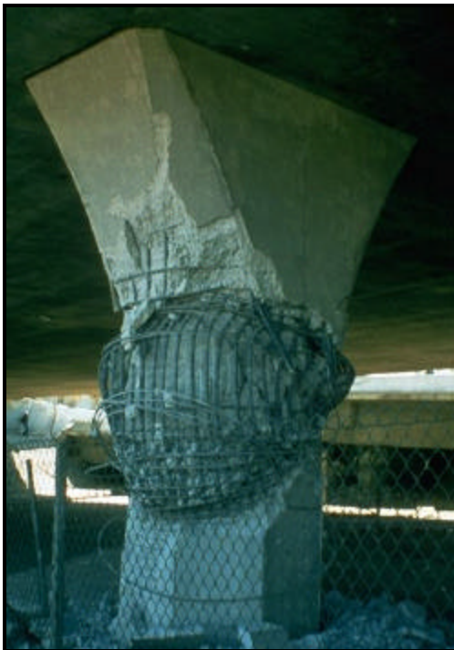
FIGURE 3.23 Column failure (11)
