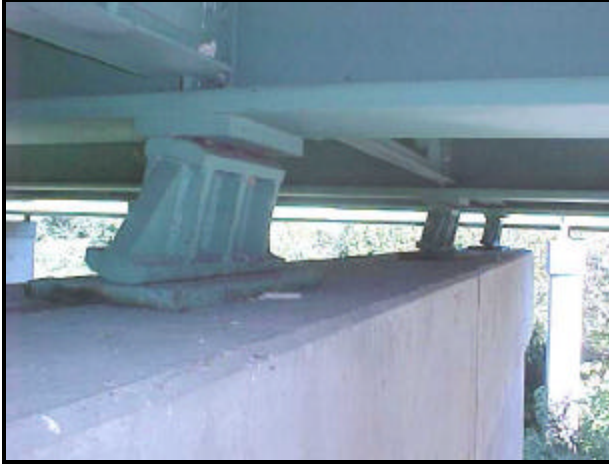
FIGURE 3.54 Tilted rocker bearings (9)
