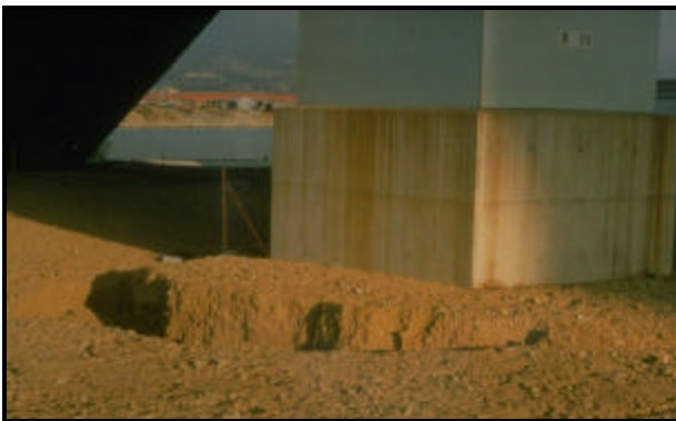
FIGURE 3.79 Settlement around RC bridge pier (11)
