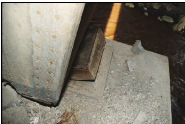
FIGURE 3.37 Failure of an elastomeric bearing due to longitudinal movement of girder (10)
