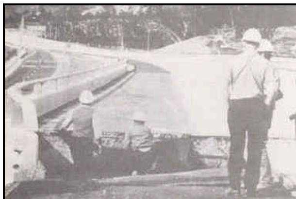
FIGURE 3.14 Excessive differential settlement of the backfill (1)
