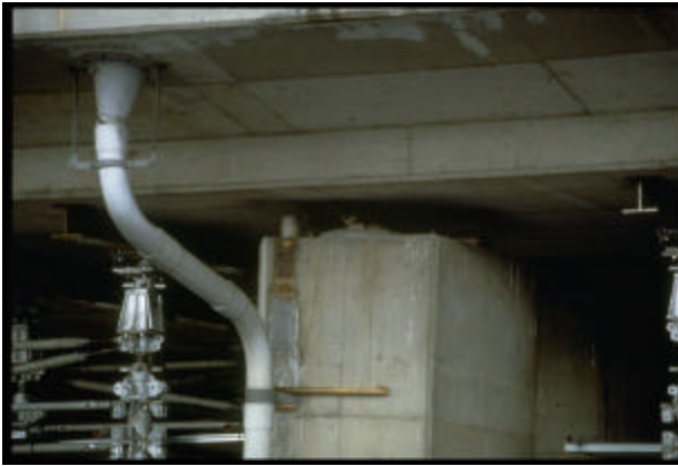
FIGURE 3.55 Shift of bearings after collapse (11)
