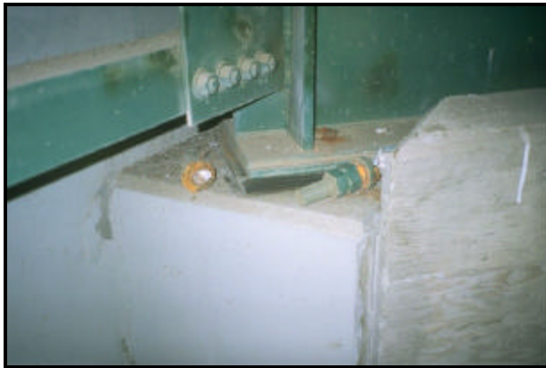
FIGURE 3.36 Failure of two anchor bolts for a girder after Northridge EQ 1994 (11)
