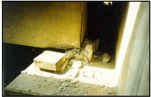
FIGURE 3.58 Sliding of elastomeric bearing (10)
