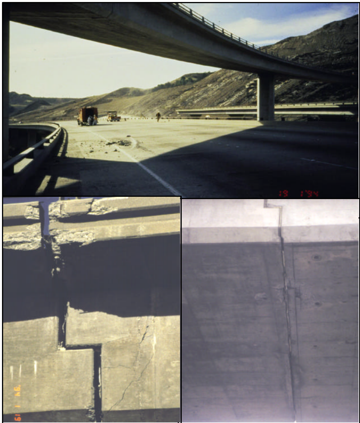
FIGURE 5.17 Different views from the superstructure of the bridge (11)
