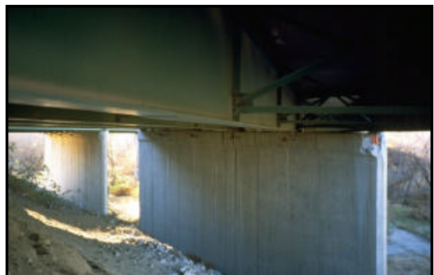
FIGURE 3.40 Spalling near location of anchor bolts after Northridge Earthquake 1994 (11)
