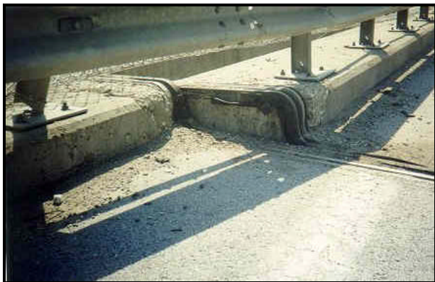
FIGURE 3.12 The excessive transversal movement of bridge after Izmit EQ (10)
