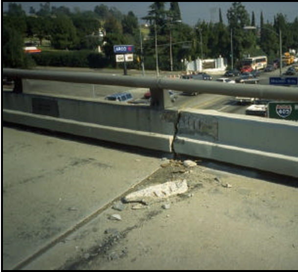
FIGURE 3.45 Minor damage on the deck of a bridge after Northridge EQ 1994 (11)
