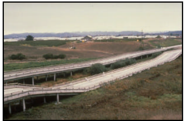
FIGURE 3.8 Collapse of RC girder bridge after Loma Prieta EQ 1989 (11)
