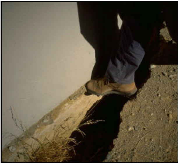
FIGURE 3.42 Separation of column from the surrounding soil after Northridge EQ 1994 (11)
