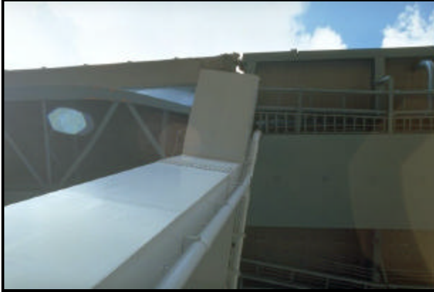
FIGURE 3.31 Buckling of steel girders (11)
