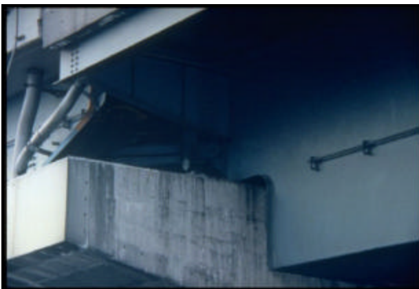
FIGURE 3.64 Steel box girder movement and collapse of bearings (11)
