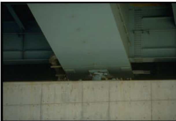
FIGURE 3.56 Bearing movement (11)
