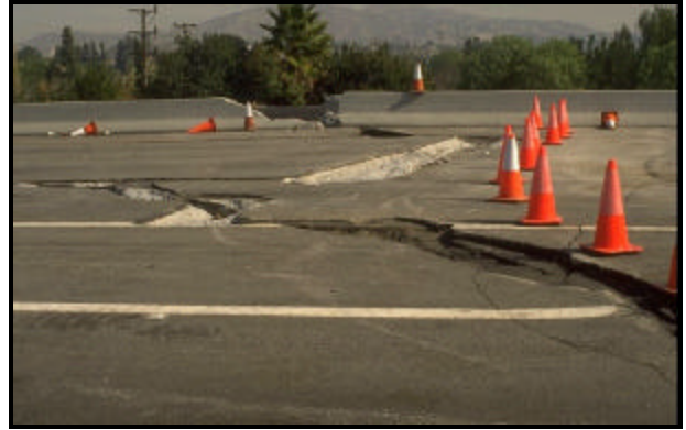
FIGURE 3.48 Surface damage to highway pavement after Northridge EQ 1994 (11)
