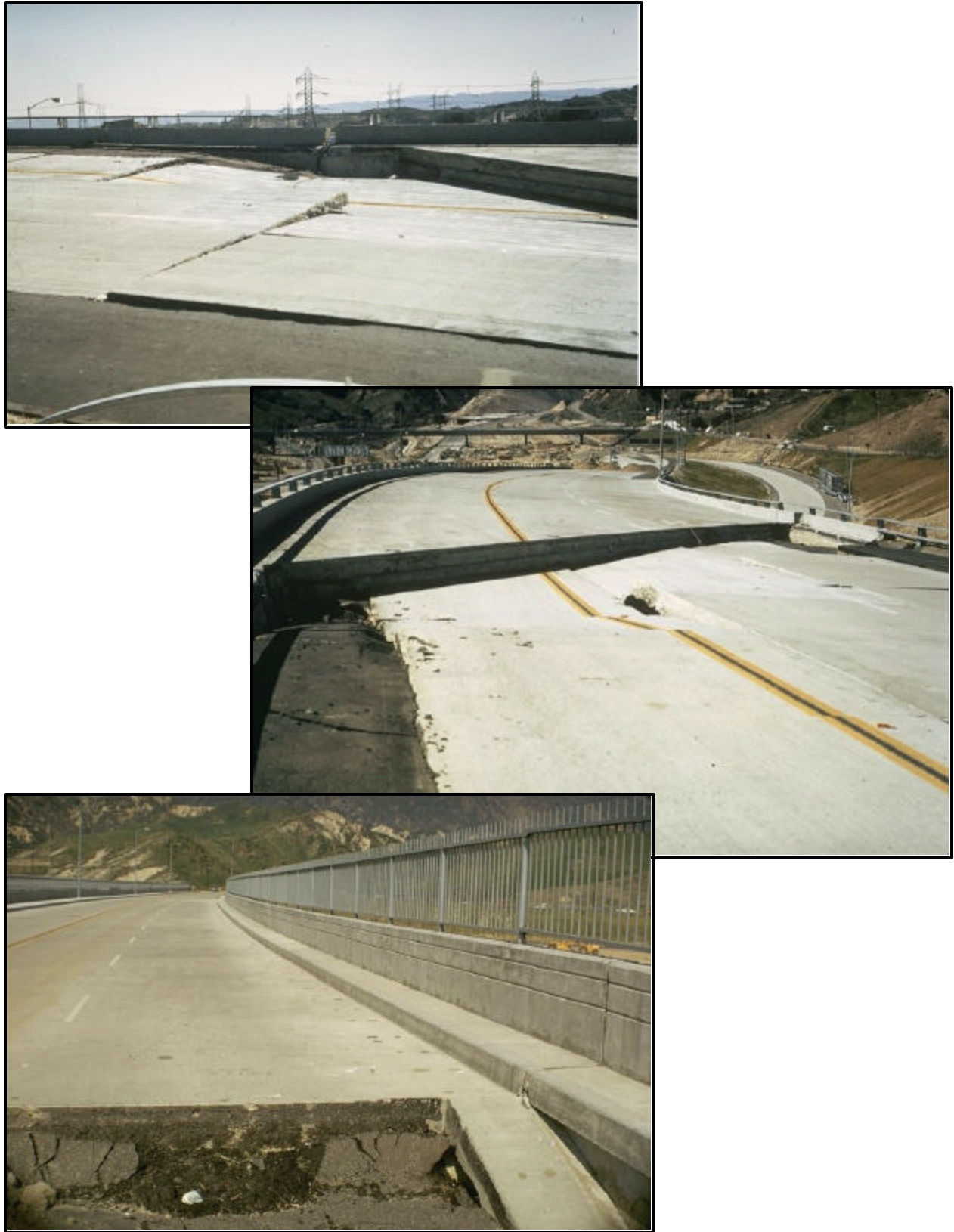
FIGURE 5.14 Superstructure damage of the third example bridge after earthquake (11)
