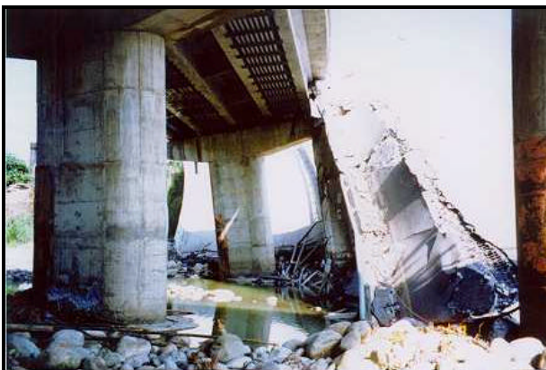
FIGURE 3.6. Collapse of deck and piers after Taiwan Earthquake 1999 (15)
