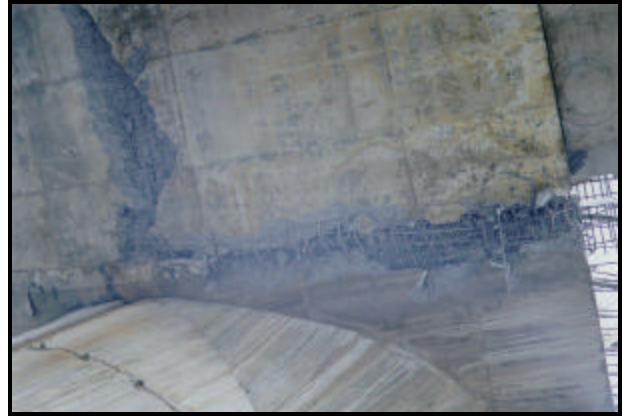
FIGURE 3.65 Heavy damage in RC box girder bridge (15)
