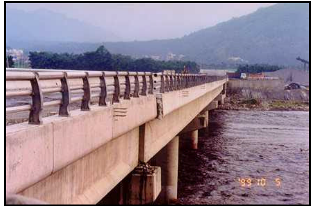
FIGURE 3.51 Transversal movement of bridge deck after Taiwan EQ (15)
