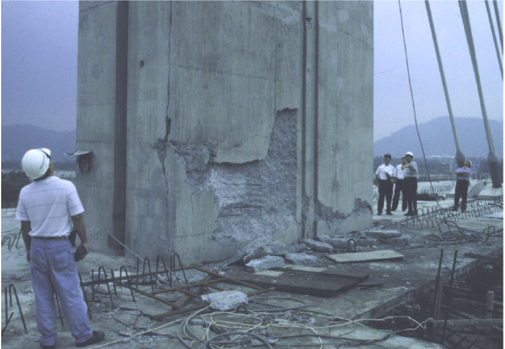
Cable-Stayed Bridge, 1999 Chi-Chi Eq. (M.O. Eberhard)
