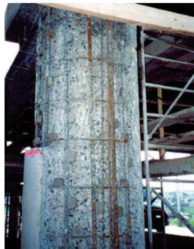
Galvashield® XP+ anode (above) Euclid Sentinel-GL (below)
