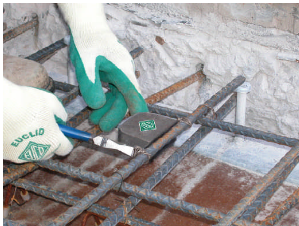
Galvashield® XP+ anode (above) Euclid Sentinel-GL (below)
