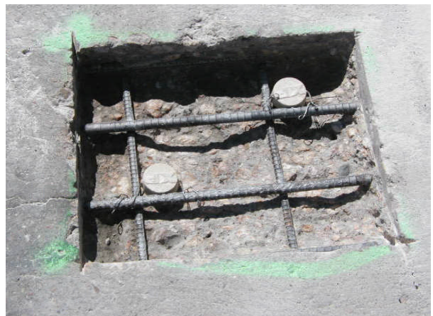
Galvashield® XP+ anode (above) Euclid Sentinel-GL (below)
