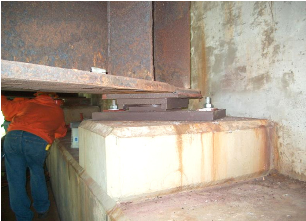
Install new bearing and anchor bolts.
