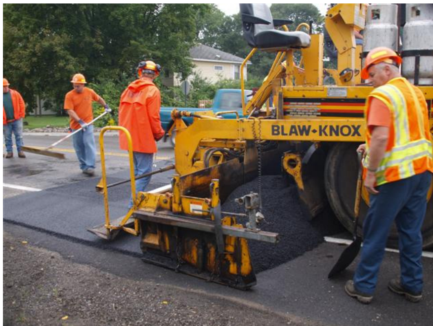
Place and compact the new asphalt wearing surface.
