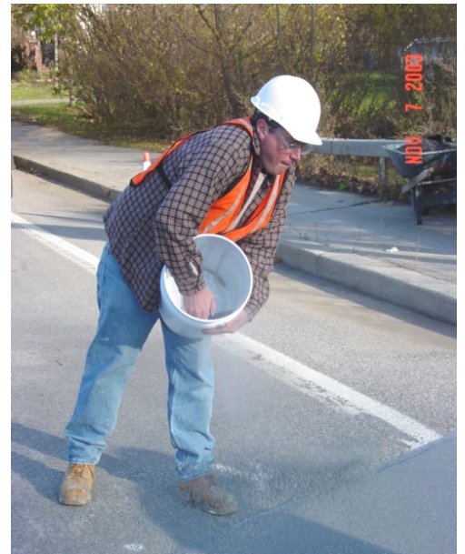
Placing Aggregate
