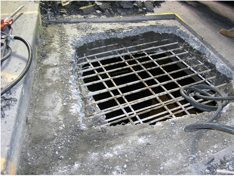
Top of Deck Repair Area
