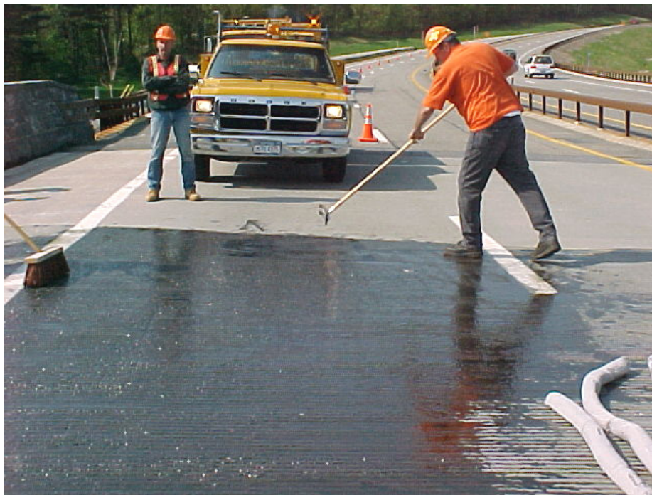
Typical application of two part “healer/sealer”.
