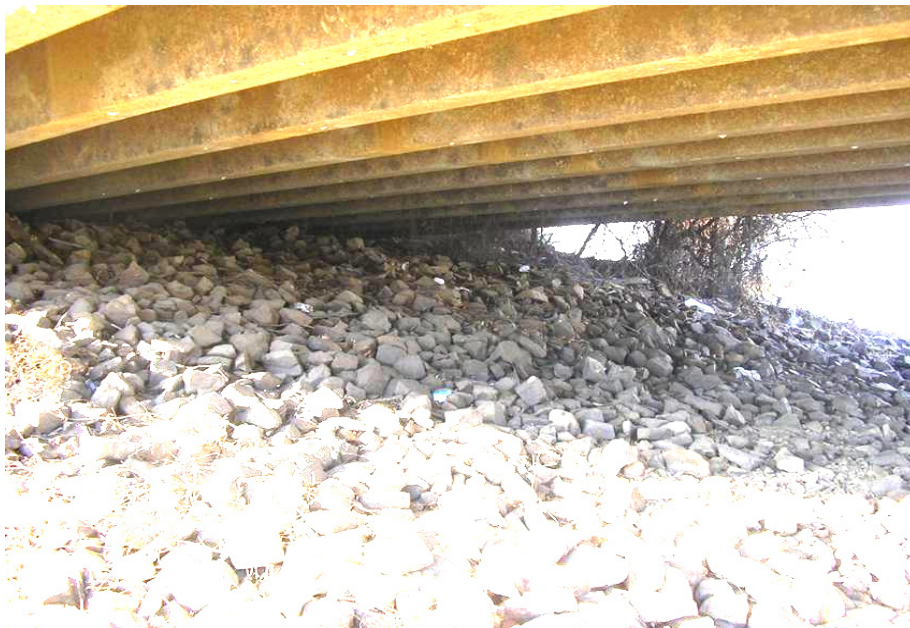
Rip-rap placed for protection of foundation and channel bank.
