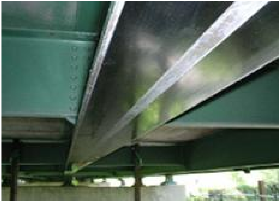
Steel properly prepared for painting.
