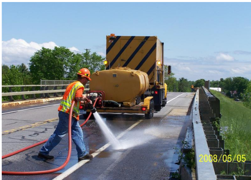
Volume washing the bridge deck.
