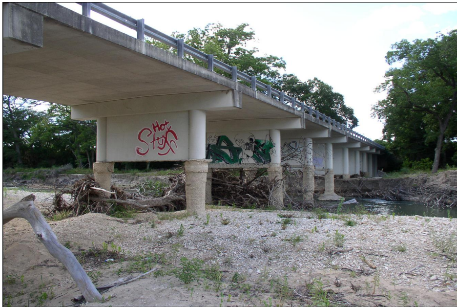
A scour incident encountered under a pier supported by drilled shafts.
