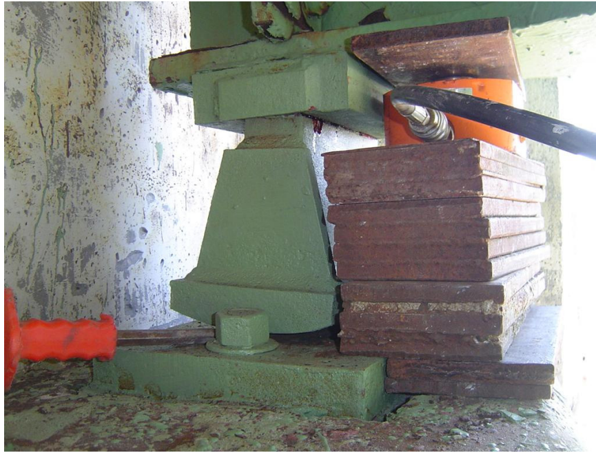
Typical bridge jacking for access to grease bearings.
