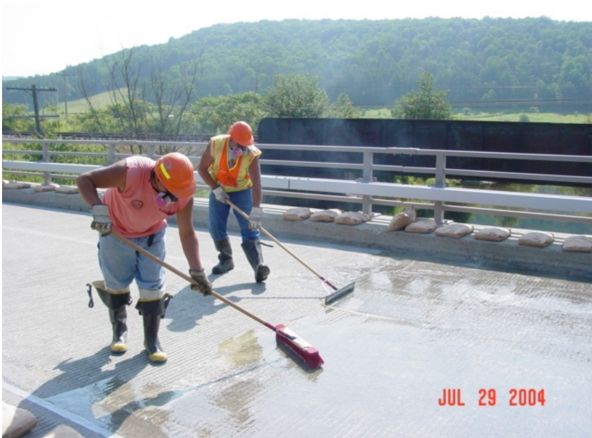
Spreading the polymer material
