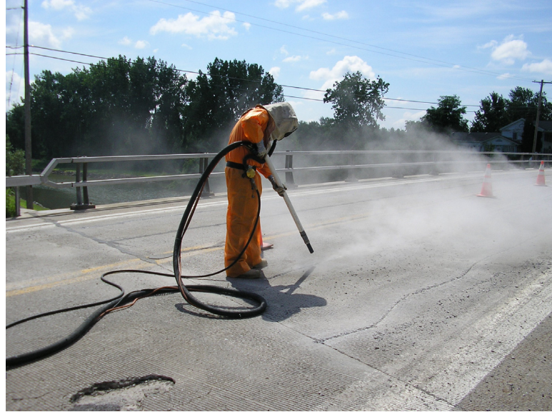
Blast Cleaning Routed Crack
