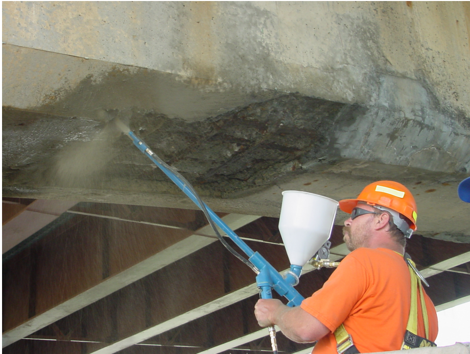
Shooting material for overhead repair
