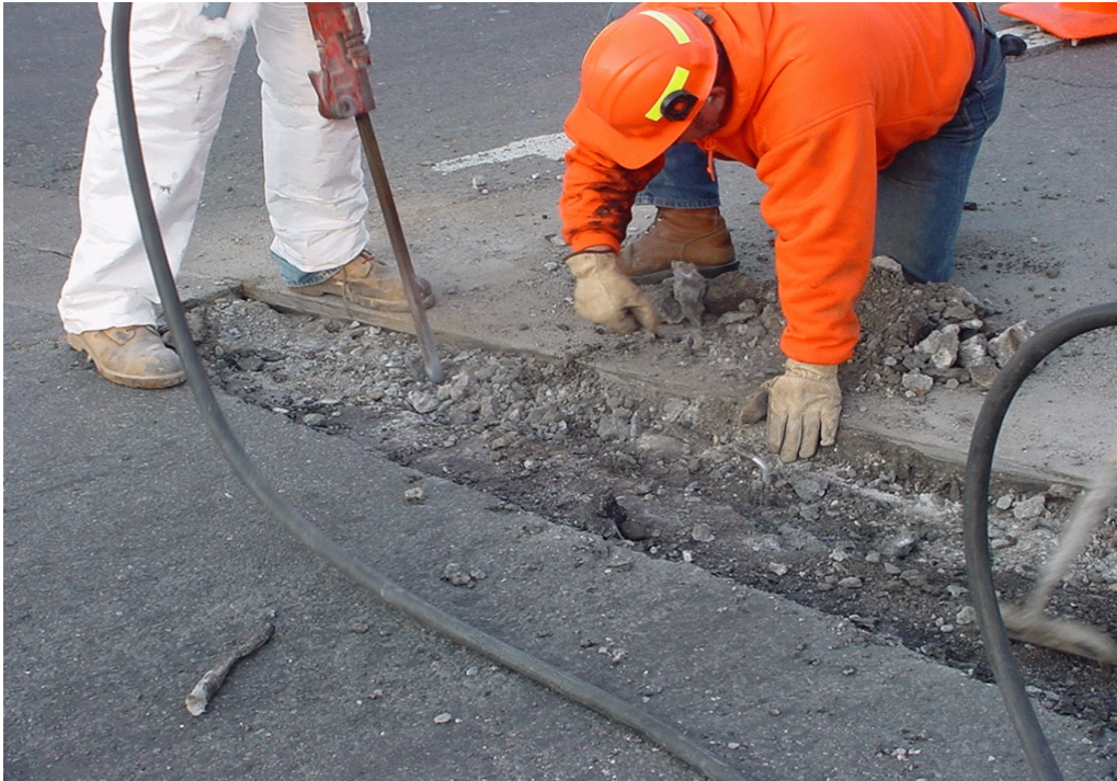
Removing concrete adjacent to the joint.
