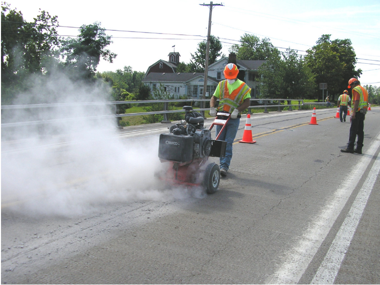
Routing Out Existing Crack
