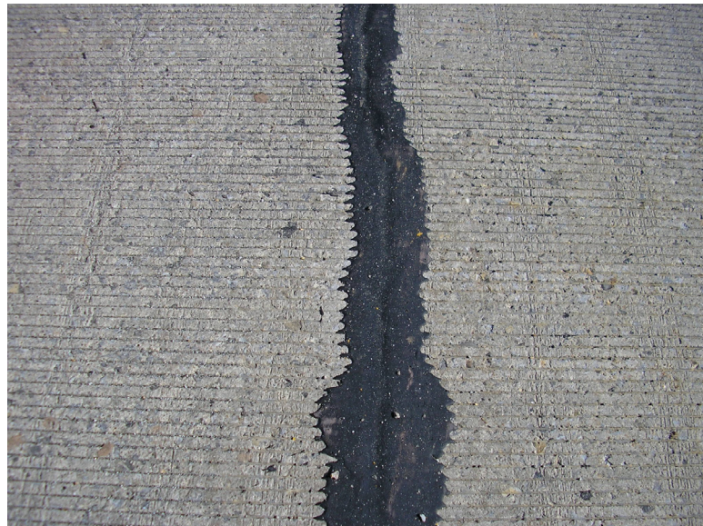
Finished Sealed Crack
