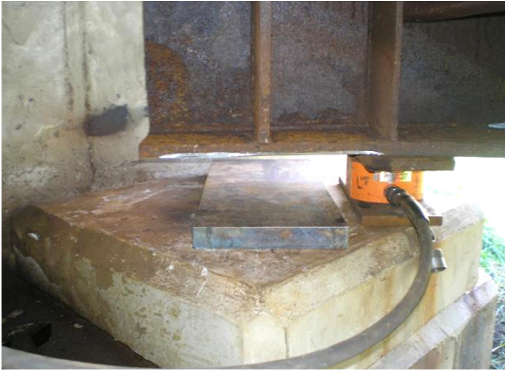
Remove existing bearing.
