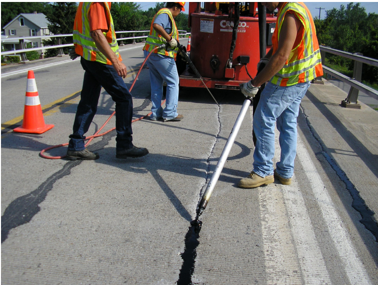
Sealing of Crack
