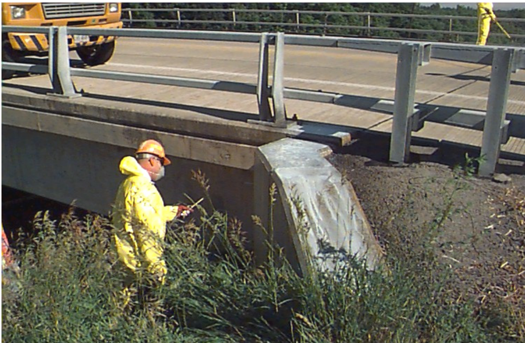
Applying penetrating sealer.
