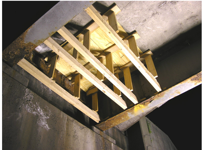
Repair Form - Bottom View
