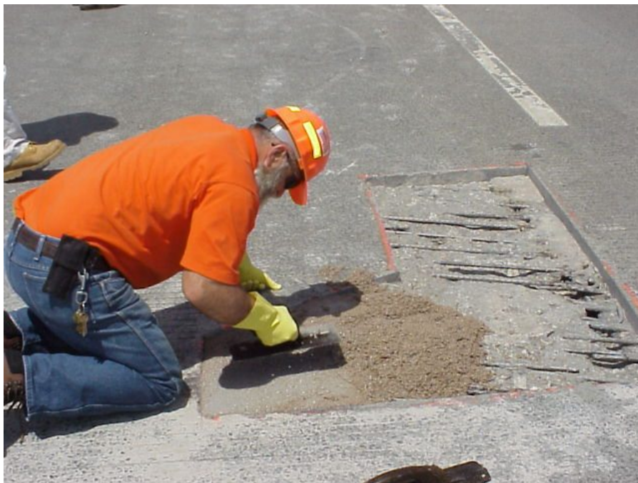
Placing repair material.
