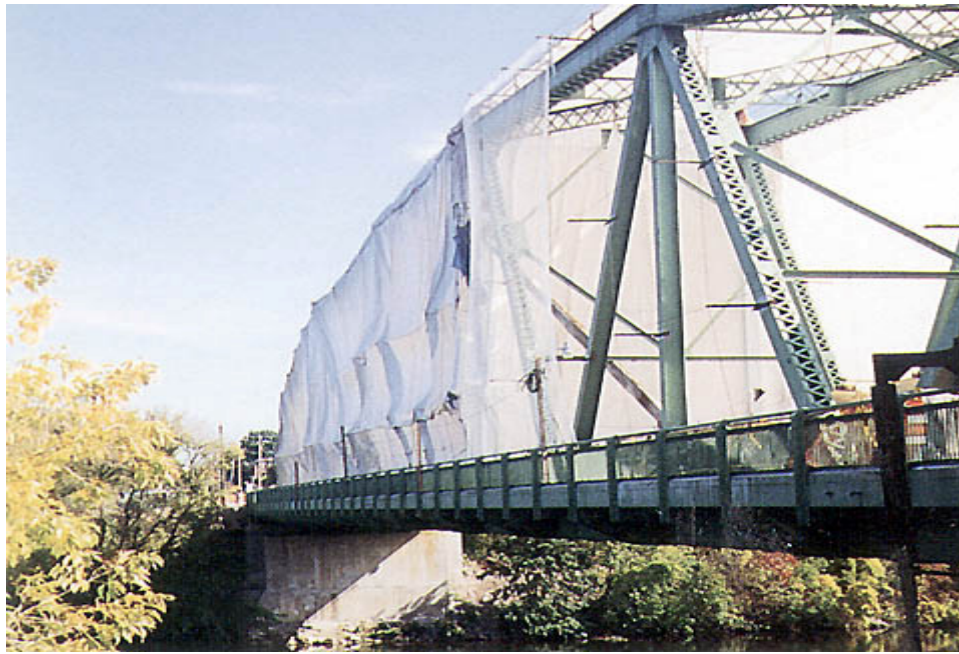
Typical paint project with Class A containment.
