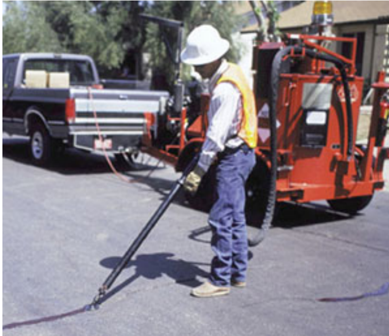
Typical crack-filling equipment and setup.
